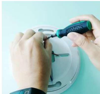
(4)Fix the hanging board with screws
